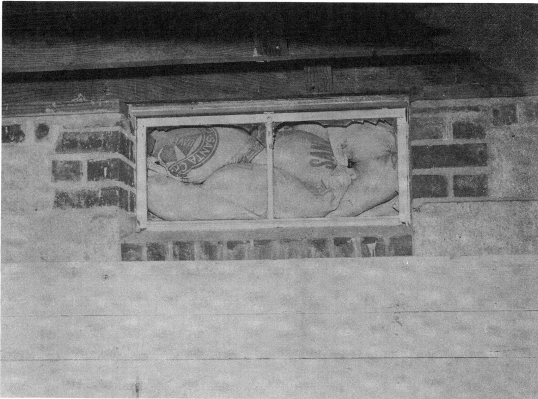
Fig. 2.23—Interior view of basement window well with sandbags in place.
